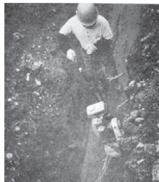
Photograph 2 A compactor helps improve efficiency
