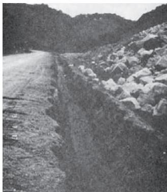
Photograph 1 Smooth out the bottom section of the trench
